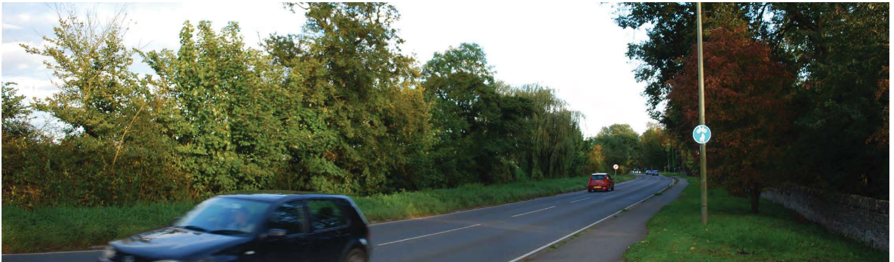
Viewpoint EW6 - Looking north east towards the Site
